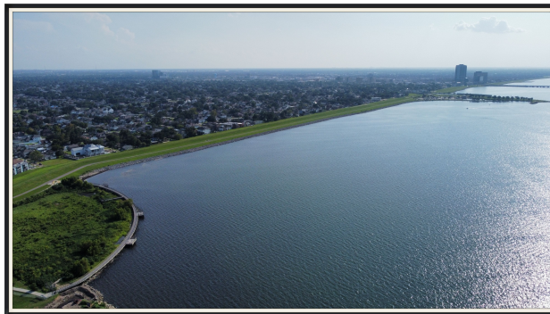
Current view from Bucktown to Bonnabel prior to rock and marsh installation.
